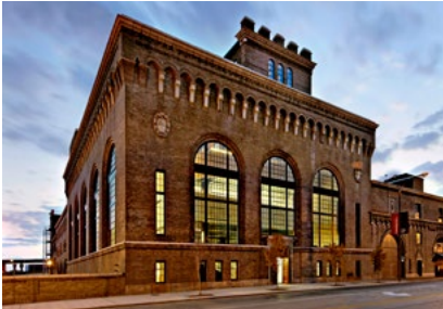
CannonDesign Regional Offices Power House Restoration/Renovation St. Louis, MO
